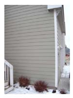
**Description:** Cement board siding nailed to the buildings' substrate with trim in regular widths, window and door perimeters, soffits and facia.
