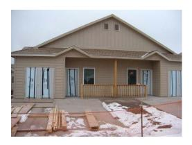
**Description:** Cement board siding nailed to the buildings' substrate with trim in regular widths, window and door perimeters, soffits and facia.
