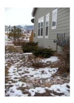
**Description:** The buildings drainage system utilizes surface slope to route stormwater runoff away from the building foundation system and into the overall site drainage system.
